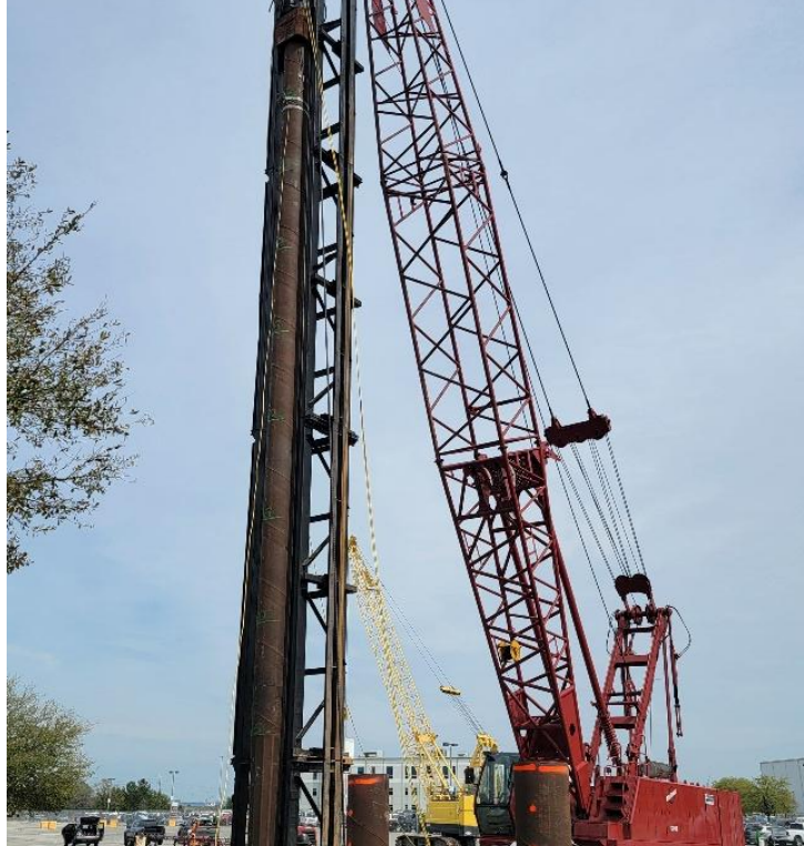
Figure 3. Tapered pile driving with PDA monitoring
